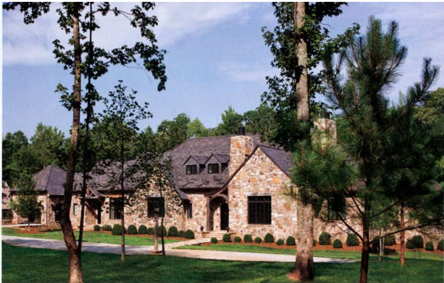
ABOVE: Tennessee fieldstone and antique Cherokee stone for facade. Marvin Windows and Doors. Chimney pots by Superior Clay Corporation. Vermont black slate on roof. BELOW: On garage, pressure-treated cedar roof. Metal columns from AP Iron Design Inc. OPPOSITE: Oak timber columns, beams and rafters, all from Wyatt Childs, Inc. Custom cypress handrails. Lanterns by David Addenbrooke Designs. Doors by Marvin Windows and Doors.
