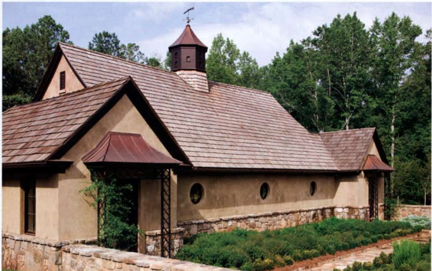
ABOVE: Tennessee fieldstone and antique Cherokee stone for facade. Marvin Windows and Doors. Chimney pots by Superior Clay Corporation. Vermont black slate on roof. BELOW: On garage, pressure-treated cedar roof. Metal columns from AP Iron Design Inc. OPPOSITE: Oak timber columns, beams and rafters, all from Wyatt Childs, Inc. Custom cypress handrails. Lanterns by David Addenbrooke Designs. Doors by Marvin Windows and Doors.
