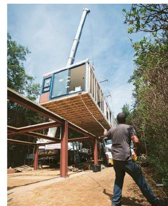
Left to right: The 2015 North Fork Bay House is a lifted double-wide/courtyard hybrid, elevated on a steel frame for flood control. A weekend house for two generations, the 1,650-square-foot open plan also tucks in three bedrooms and two and a half baths.
