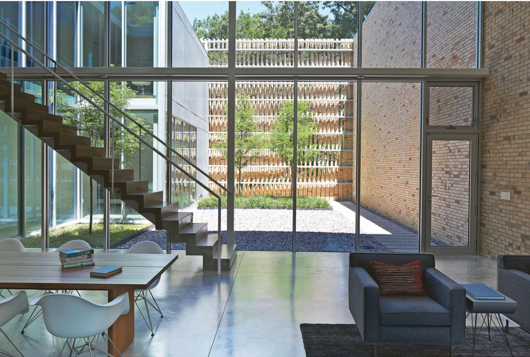
*This page:* The permeable wall permits natural light to penetrate the interiors during the day, and allows for the interiors to project illumination through the street façade at night. The brick becomes a solid wall on the east side of the courtyard, flanking the entry path and moving past the glass-front façade, through the great room, and out to the rear yard.
