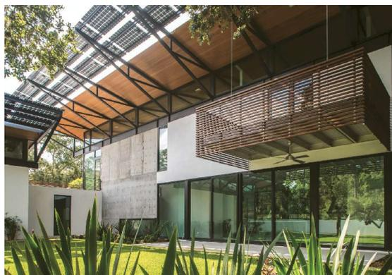
Far left and left: Custom steel trusses suspend a balcony in the design/build Seminole Residence. Generous overhangs and a courtyard plan create a protected microclimate for outdoor living.
