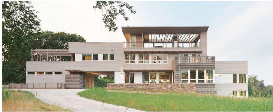
Above: The 2012 Fishers Island House required ferrying modules from the mainland to the island. So, RES4 turned to a system of smaller 12-foot-wide modules. The typology used here is a combination double-wide/triple-wide hybrid for a total of 8 boxes and 4,469 square feet.
