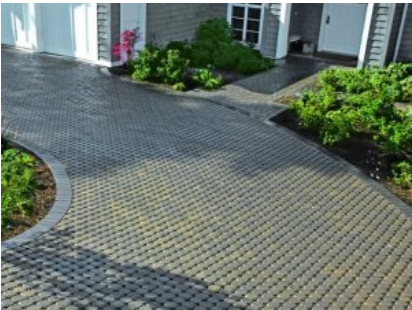
Prevent Puddles with Pervious Paving Materials
